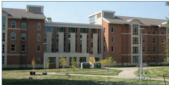
Exterior walkways to residence halls
