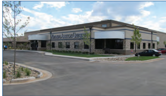
Exterior of the new $4 million campus
