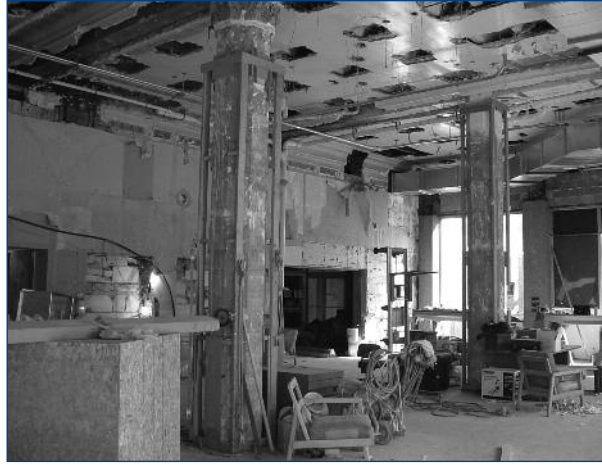
Work underway in one of the 46 apartments in the building.
